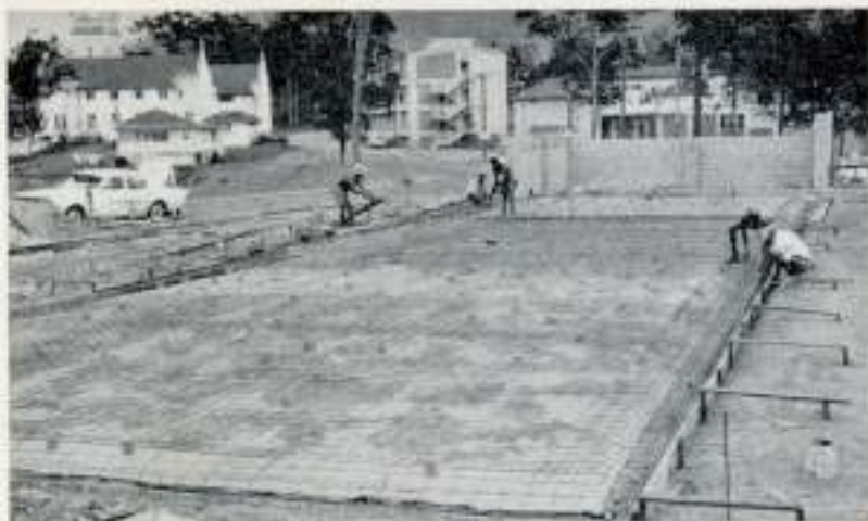
Floor ready for concreting
