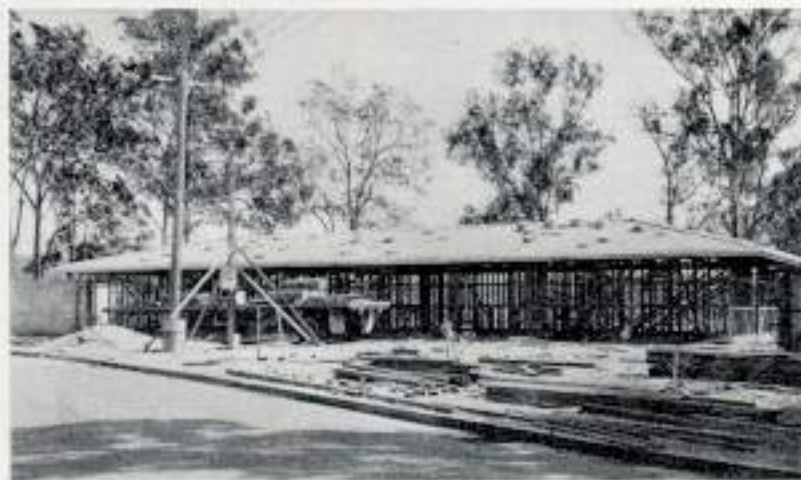
The Building rises.
